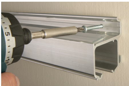
Step 1: Install wall-mount track.
